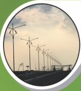
Street and Highway Lighting
